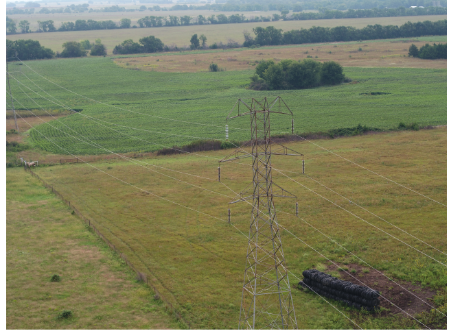
Figure 2: An example of a power-line image.
